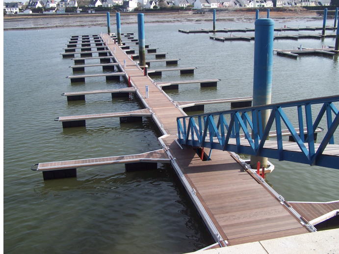
Pontons flottants - Port-Louis (France)
